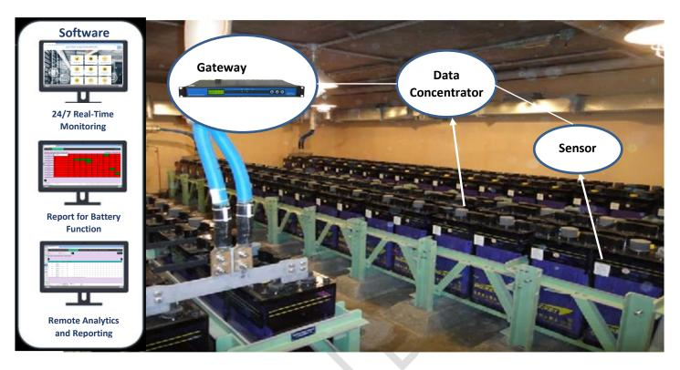
T-BMS-300 Battery Monitoring System assure the performance of the backup battery power system, it will also reduce UPS battery maintenance and replacement cost. Ineffective and expensive manual testing on a quarterly basis can be eliminated. With a T-BMS-300 system, battery replacement decisions are based on data and predictive analytics rather than fear of failure. As a result, battery life is extended by up to 65%.
