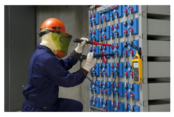
Generally, all datacenters will have huge capacity of battery banks cascaded with huge number of individual batteries to maintain power source, in existing setup it is very difficult for an operator to check and monitor the voltage, current and other parameters of each battery in a battery bank. Currently operator has to measure with the help of multimeter across individual battery.
